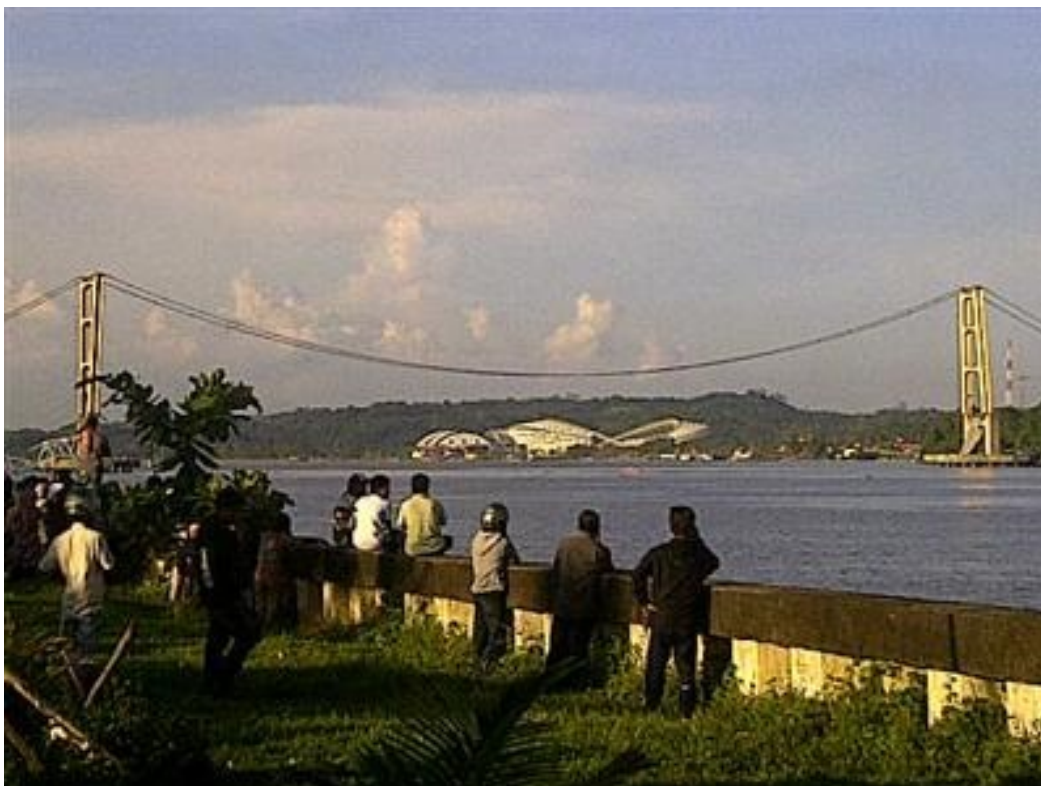
Photo 1 Kukar Bridge before collapse (Source IN, some signs of collapse are visible)
